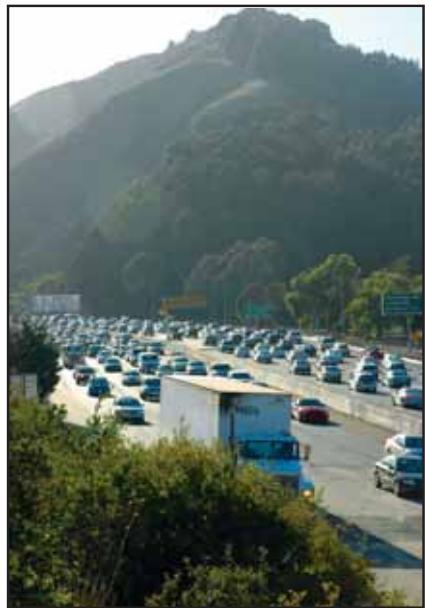
SALLY HOGARTY Congestion leading to and from the Caldecott Tunnel may not ease if funding is pulled on the proposed fourth bore.
